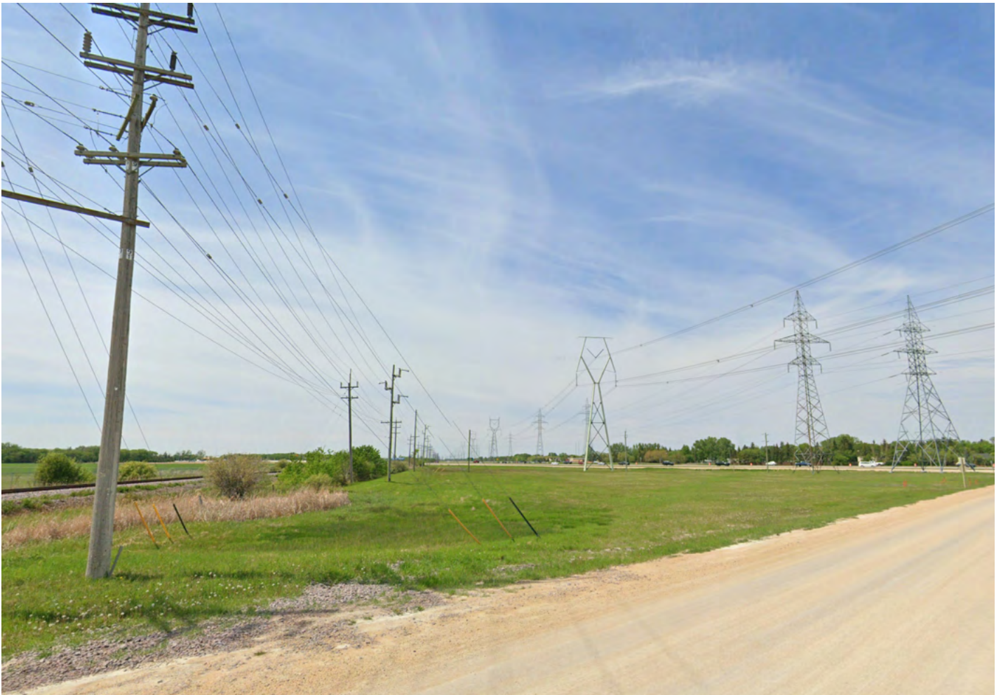
Figure 8. Manitoba Hydro Transmission Lines
